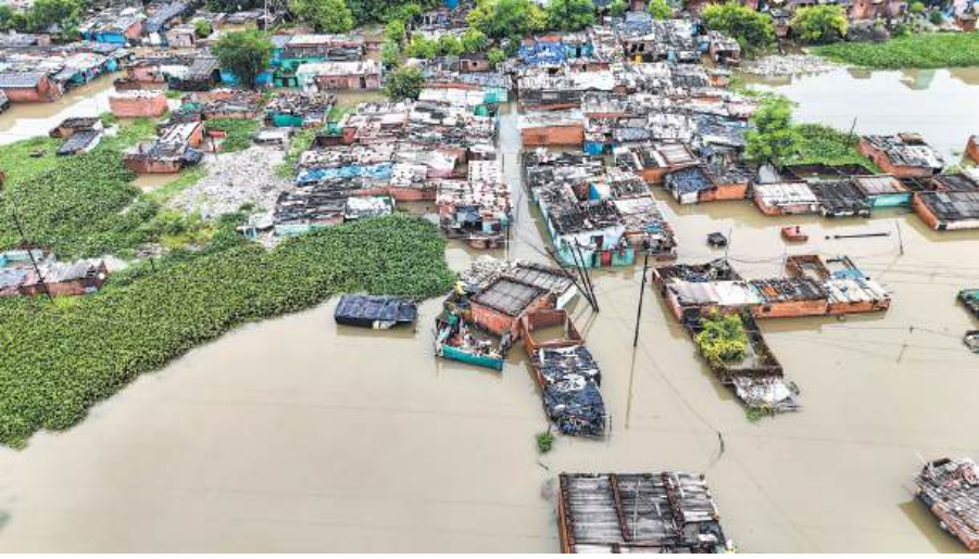
An aerial view of a residential area partially inundated after heavy rainfall and subsequent rise in the Pandu River water level, in Kanpur.
