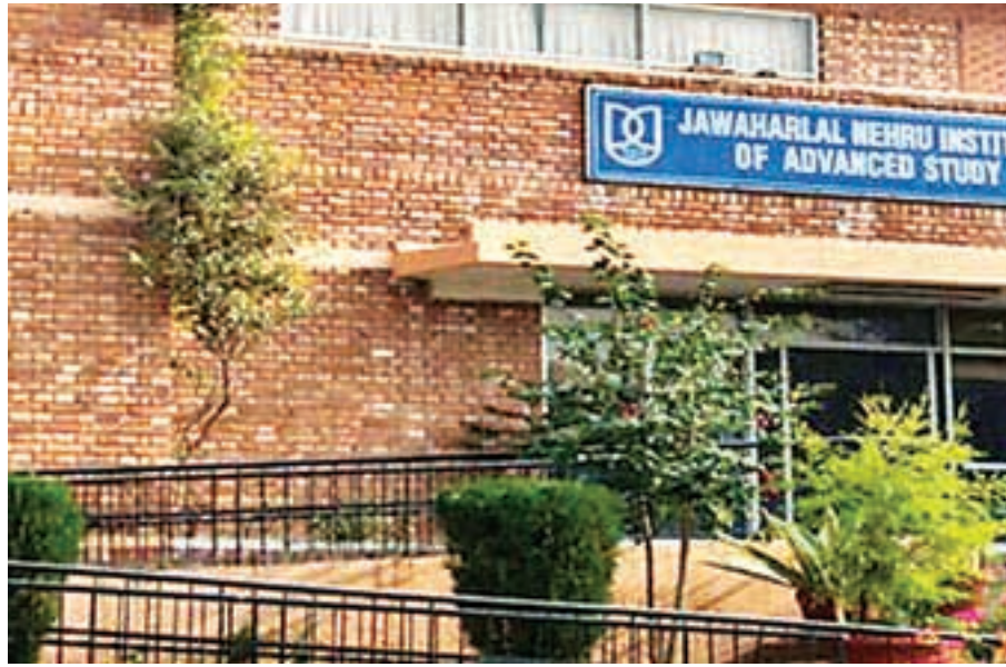
A view of JNU administrative building.
