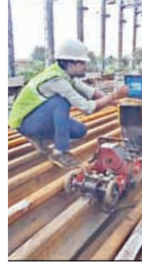
An employee working on the long rails.
