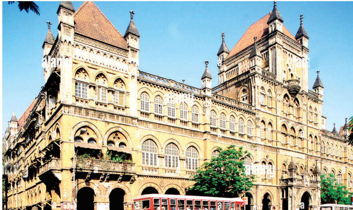
A view of Bombay High Court.
