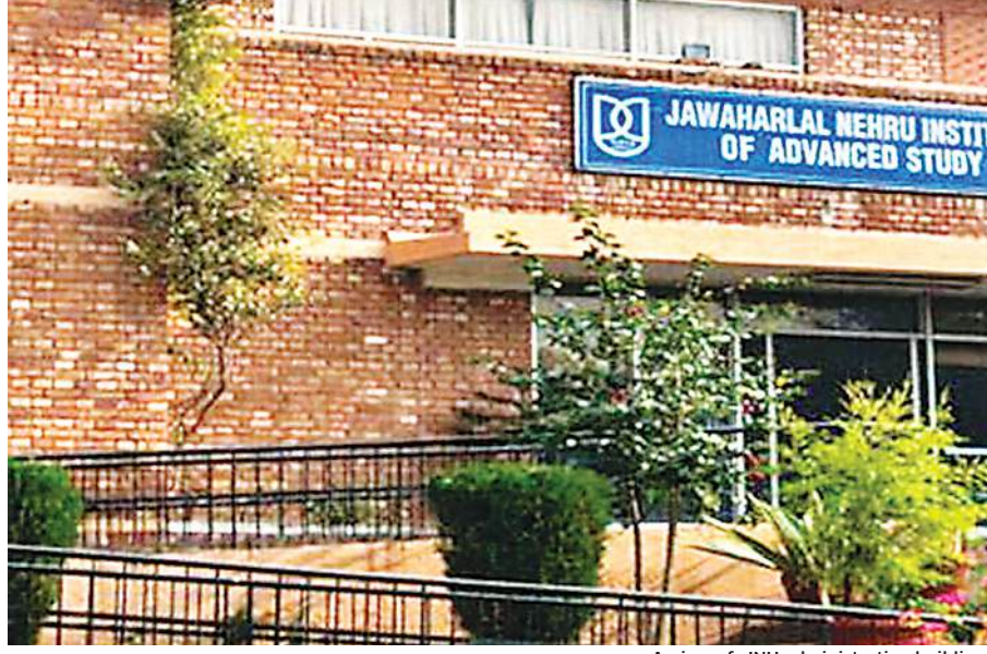
A view of JNU administrative building.
