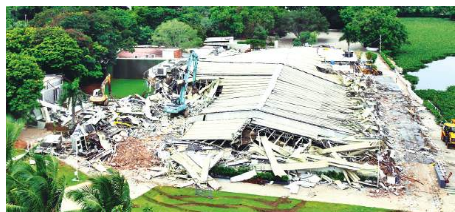
The N Convention, jointly owned by actor Nagarjuna, being demolished in Hyderabad. | Photo: PTI
