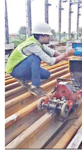
An employee working on the long rails.
