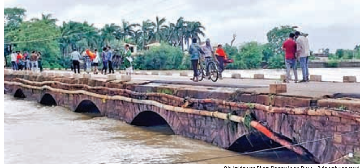
Old bridge on River Sheonath on Durg - Rajnandgaon road.
