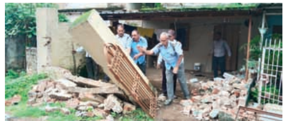
Doors and windows being removed.
