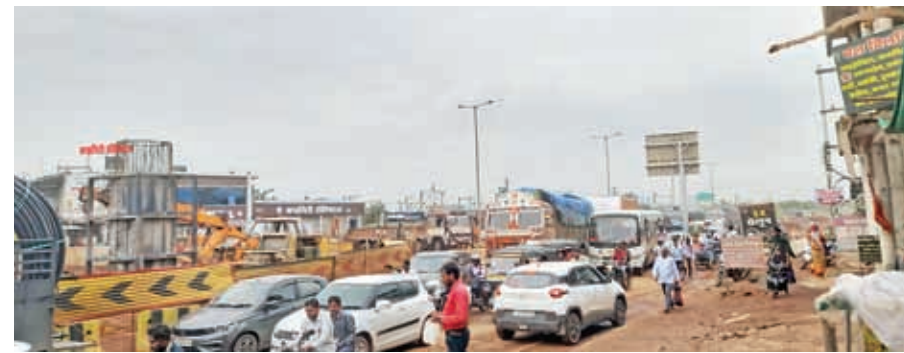
Overbridge construction causes severe traffic disruptions.
