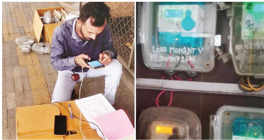
Worker installing electric meter at Kabir Nagar.
