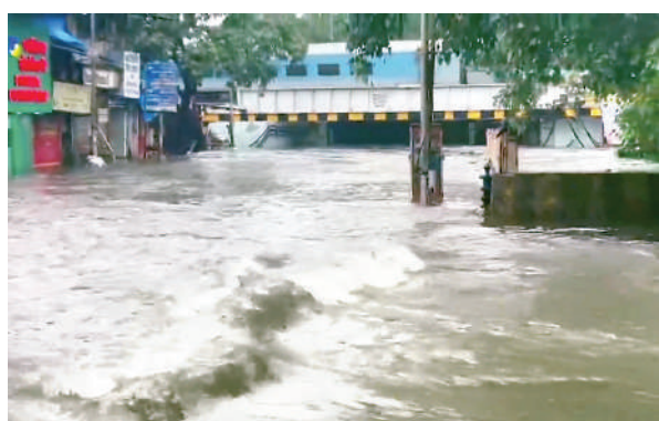
Flooded Andheri Subway following heavy rainfall, in Mumbai. | Photo: PTI
