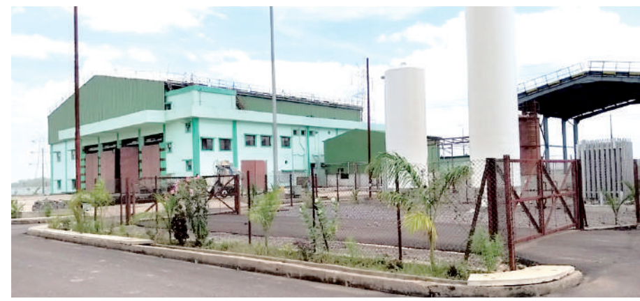
The PCB Plant at BSP is one of the largest facilities in entire South Asia.
