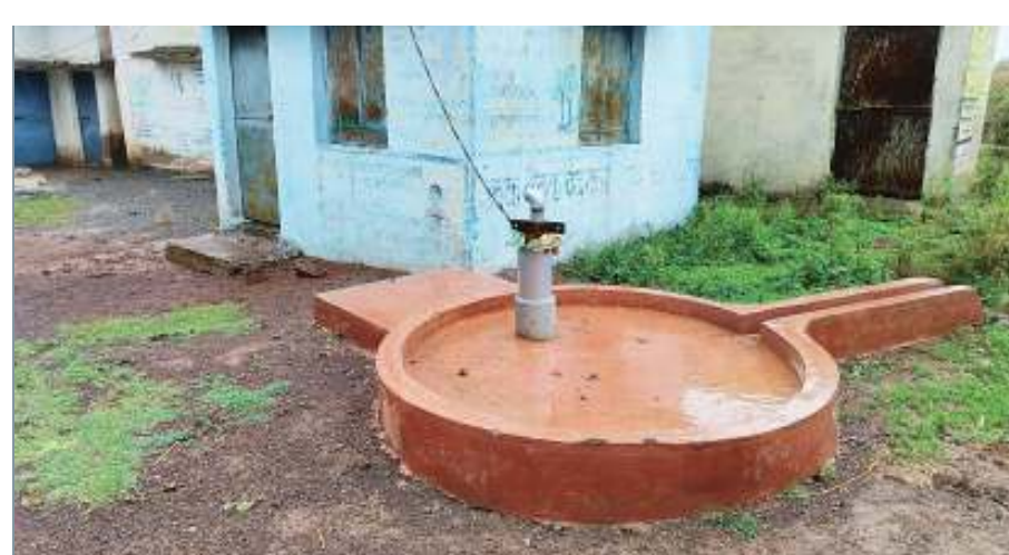
Drinking water is being supplied by installing a power pump in Pirchatola.
