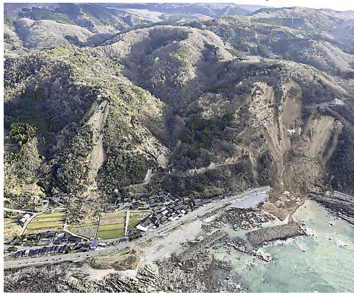
This aerial photo shows a national road is blocked by landslides caused by earthquakes in Suzu, Ishikawa prefecture, Japan Thursday, Jan. 4.
