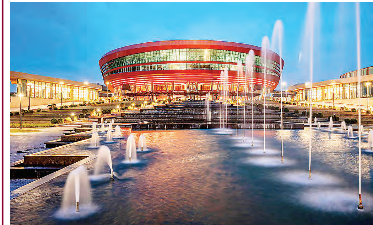
The redeveloped ITPO complex which will host the G20 leaders' meeting in September. Prime Minister Narendra Modi is likely to inaugurate the complex on July 26.
